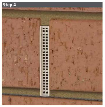
The High Performance Bushfire Weepa has a specially formulated grate (with stainless steel mesh set behind) which chars and self extinguishes.
