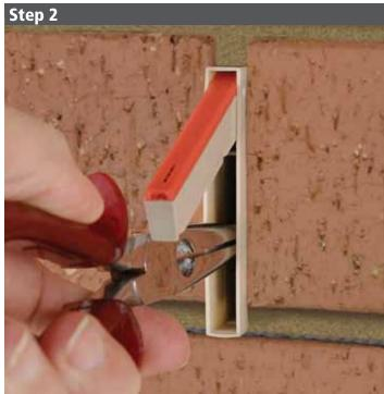
When rendering, the Weepa needs to be loosened in the masonry so the renderer can adjust the Weepa in and out. Grab internal rib to adjust Weepa in and out.
