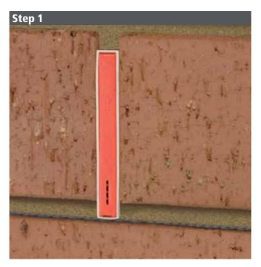
Install the Weepa between bricks or blocks, at specified intervals and firmly in contact with the flashing. For rendering, set out a few millimetres.
