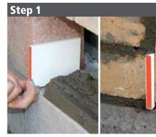
Make sure the new Weepa is installed when the masonry wall is built.
