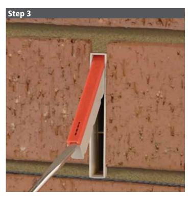
After clean up, use a small, flat screwdriver to prise the mortar cover up at the bottom.
