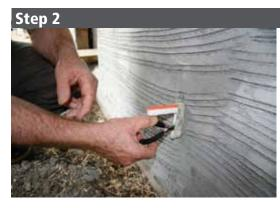
Loosen the Weepa and pull out proud of masonry.
